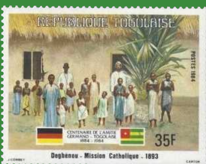
ABOVE: 35f design showing the Catholic Mission at Degbenou in the south of the country in 1893. Mission schools were the basis of the education system in Togo in the early years of the Protectorate
