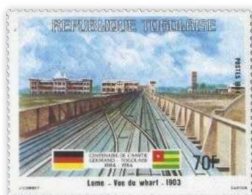
ABOVE: 70f design illustrating the wharf in Lomé in 1903, including the railway tracks which branched off from the Lomé-Aného line and, in the background, the Governor's Palace
